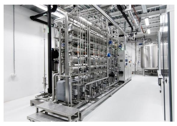
Pre-preparation; Purified water; Water for injections; Pure steam.
